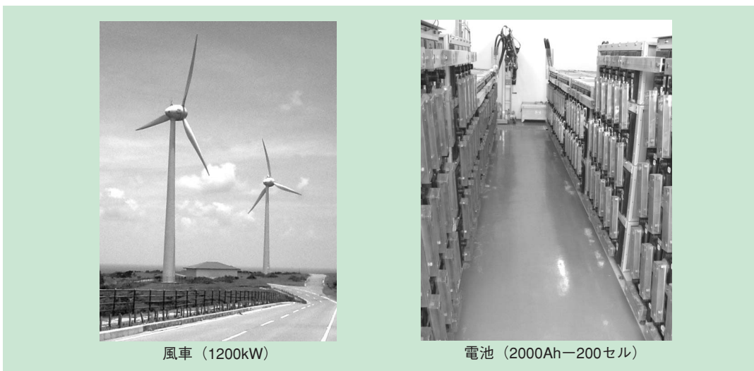
図4 風車と電池写真 Fig.4 Wind Turbine Generator and LL Type Battery.
