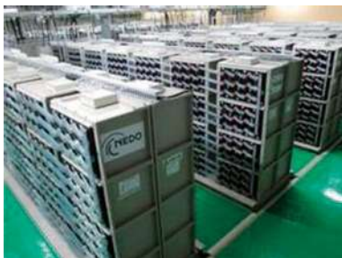
図2 伊豆大島に設置された新型鉛蓄電池設備 Figure 2 Advanced lead-acid battery systems which were installed on Izu-Oshima
